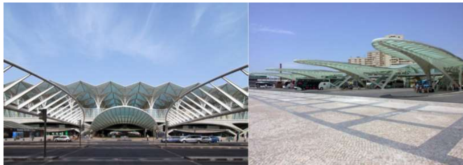
Figure 4: Gare do Oriente – Canopy Steel Structure [8]
