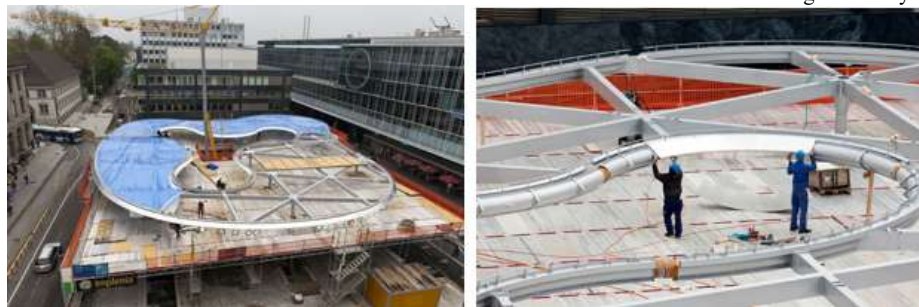
Figure 3: Aarau Bus Station – Canopy Steel Structure [7]
