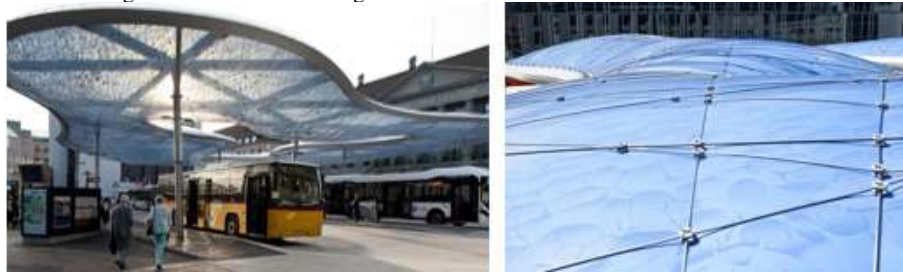
Figure 1: Aarau Bus Station Canopy and Membrane [1, 6]
