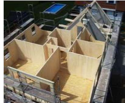
Figure 1, cross laminated timber
