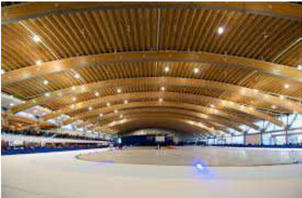
*Figure 3. Big sport hall with a roof from glued laminated beams produced based on certain design*
