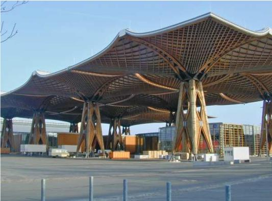
*Figure 4. Very special construction from glued laminated beams*
