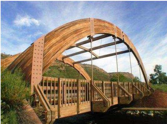
*Figure 5. Special construction of a bridge from glued laminated beams*
