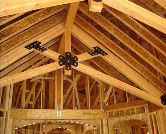
*Figure 2. Special roof construction which include different types of glued laminated beams in certain parts*
